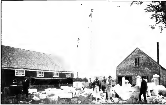
STONE SHED AND YARD OF A. F. BURTON
