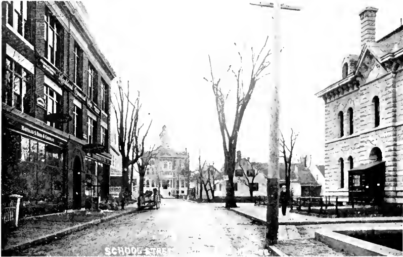
SCHOOL ST. SHOWING THORNDIKE &amp; HIX BLDG. ON LEFT
