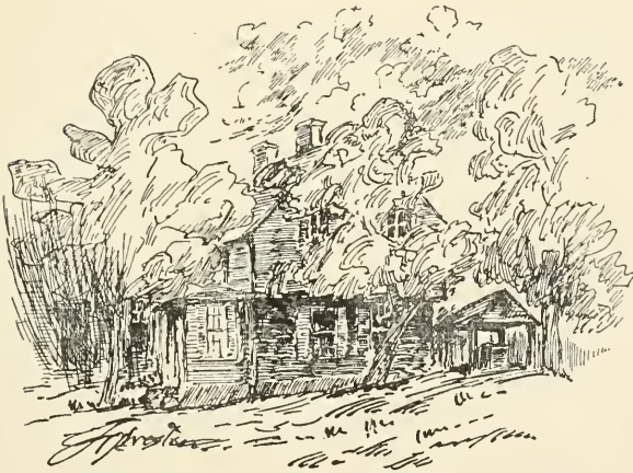
CUTT GARRISON HOUSE, KITTERY
