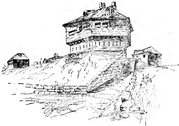
BLOCK HOUSE, FORT M'CLARY
