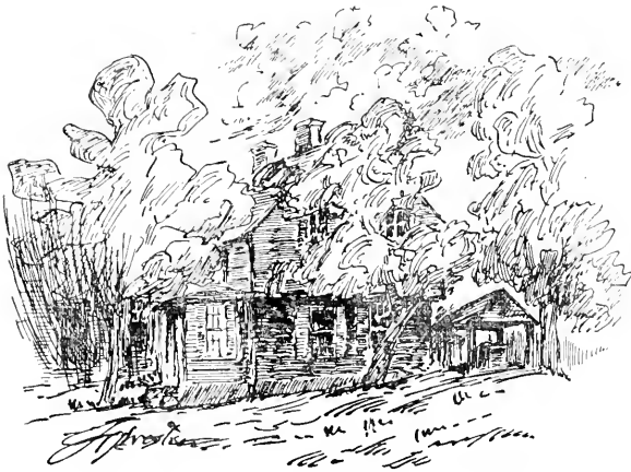
CUTT GARRISON HOUSE, KITTERY
