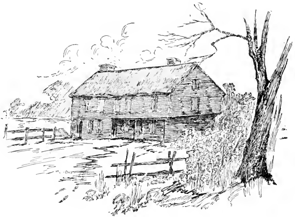
McINTIRE BLOCK HOUSE
