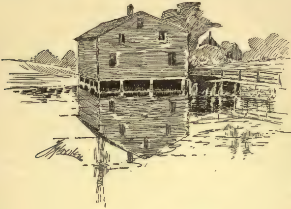
STURGEON CREEK WAREHOUSE
