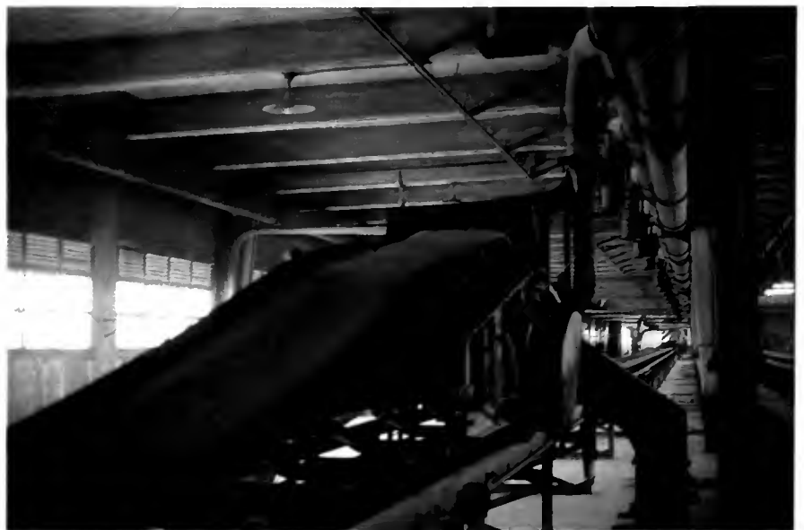
Modern export facilities using high-speed belts and bucket elevators provide efficient loading and inspection.
