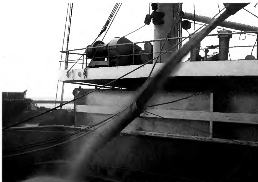
Directly under the spouting, breakage (as measured by USDA-BCFM sieves) reached 12.1 percent. Samples from the vessel clearly showed extensive breakage during loading.
