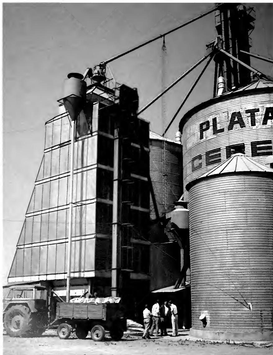
High-temperature dryers and metal storage bins provide drying and storage services for Argentine farmers
