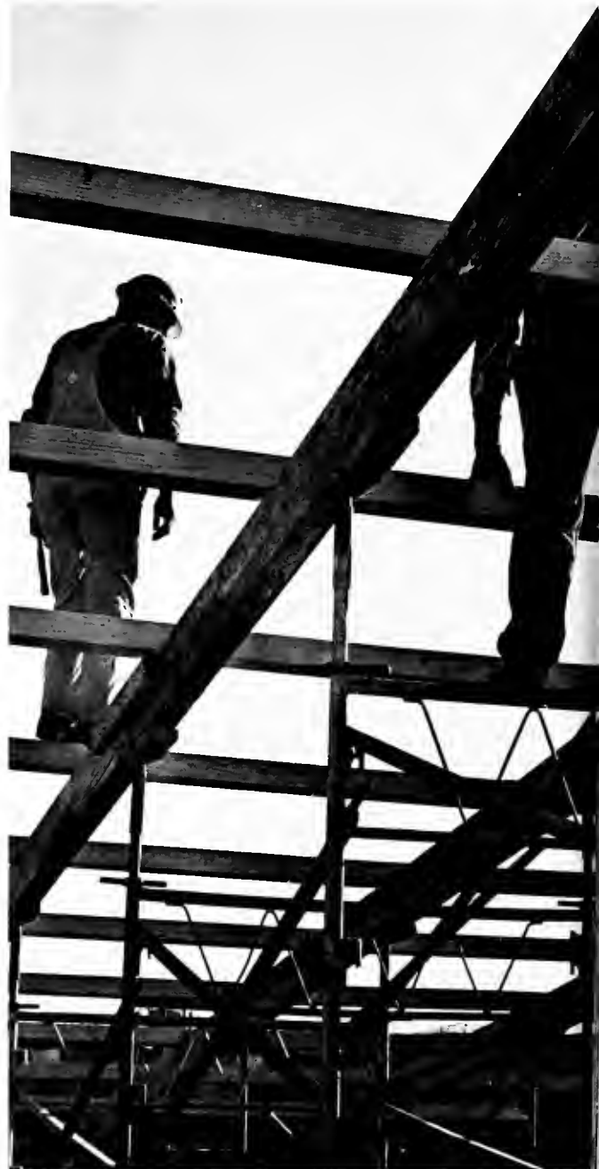
Workmen perch precariously on scaffolding.
