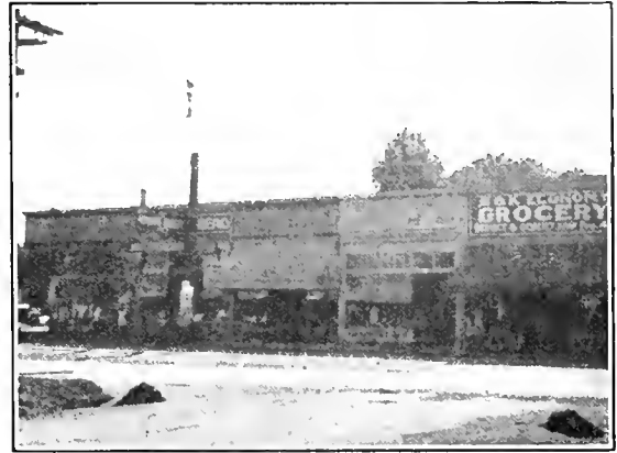
FRAME BUILDINGS TO BE REMOVED FOR ELIMINATION OF JOG AT 41ST AVENUE AND VICTORIA DRIVE. LOOKING WEST ACROSS VICTORIA DRIVE.
