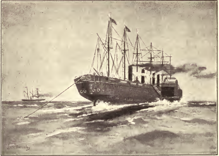
Laying the Atlantic Cable (1866)
