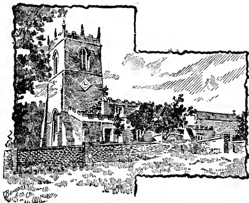
PARISH CHURCH, EPWORTH.
