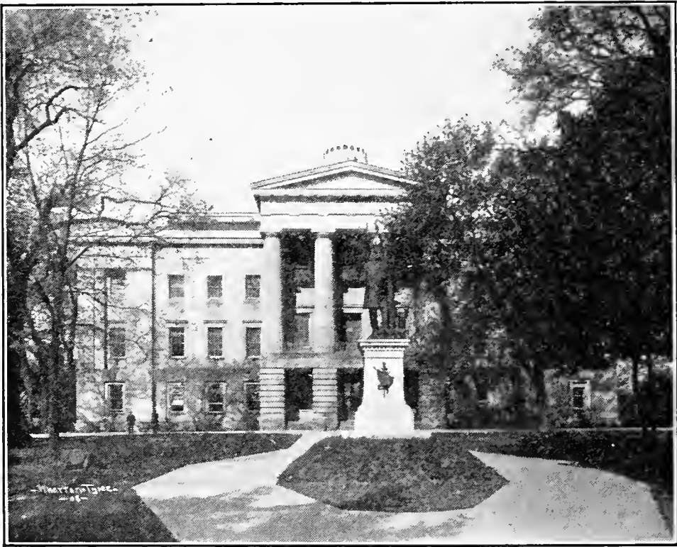
CAPITOL OF NORTH CAROLINA AS IT LOOKS TO-DAY (East front showing statue of Z. B. Vance in foreground)
