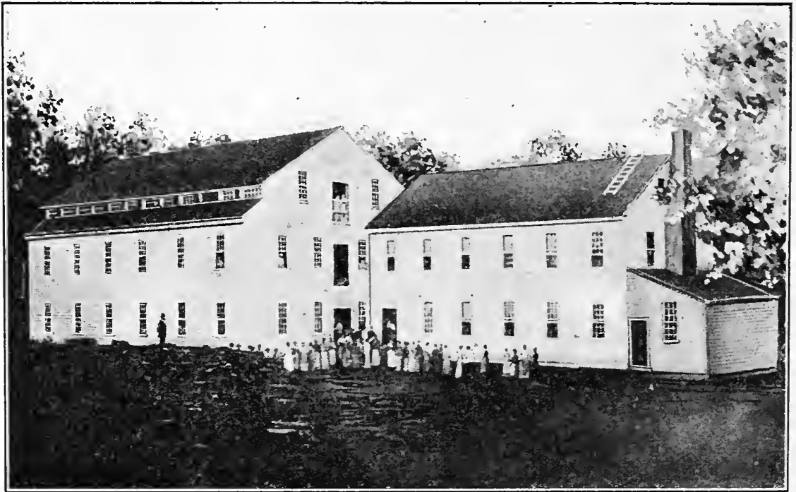
THE OLD ALAMANCE MILL, BURLINGTON, N. C.
