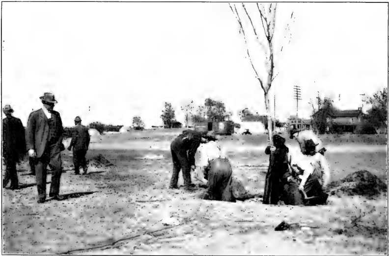
COPELAND PARK BEFORE
