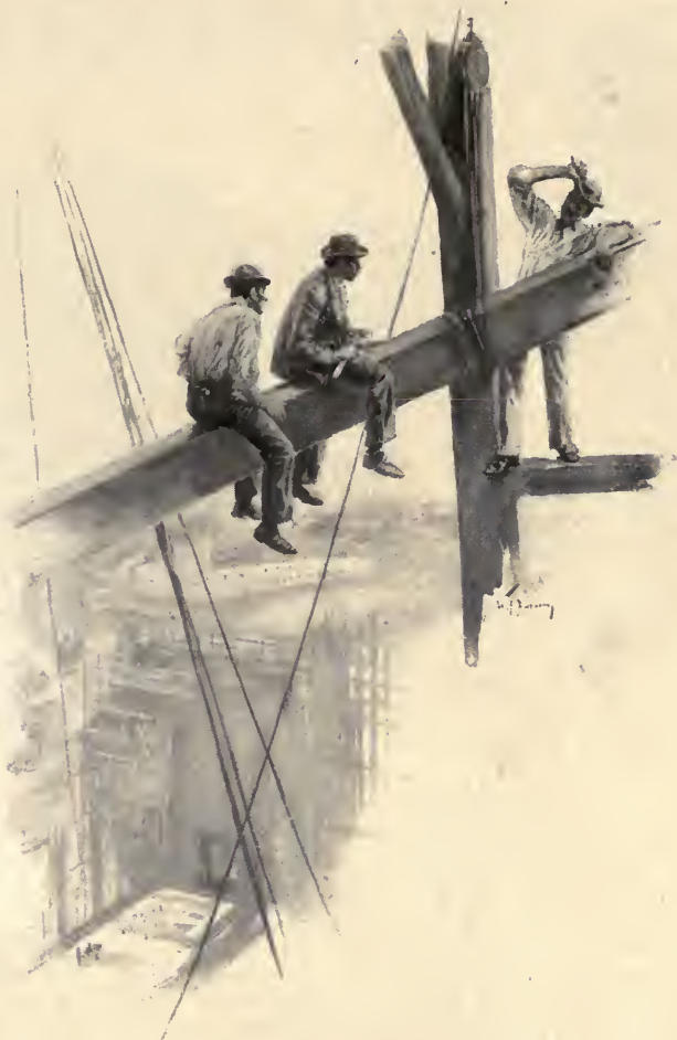
Up Among the Great Iron Arches of the Hall of Manufactures.
