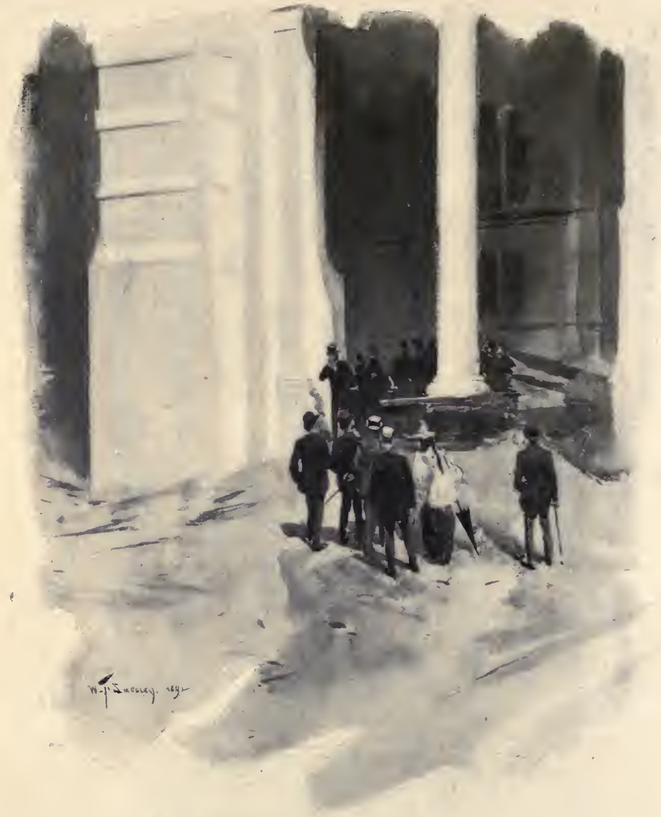
In Process of Construction (an Entrance of the Hall of Mines).
