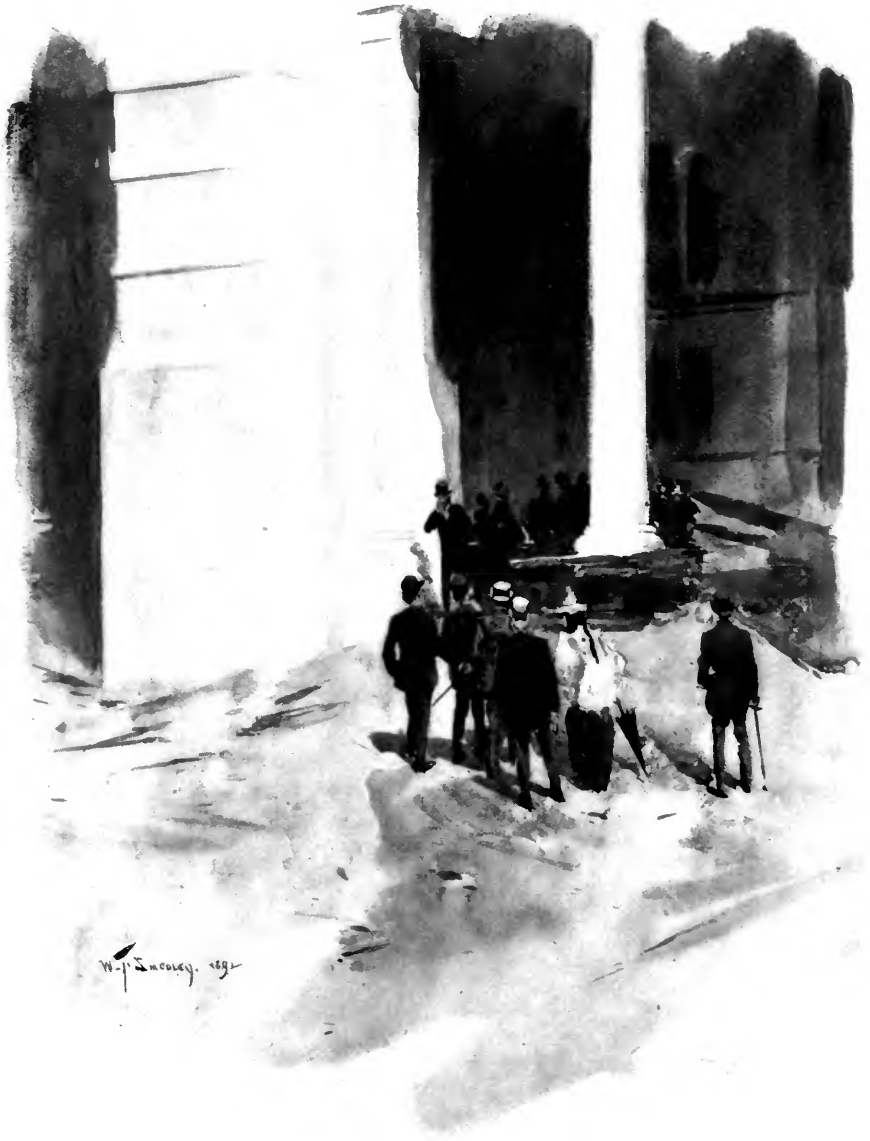
In Process of Construction (an Entrance of the Hall of Mines).
