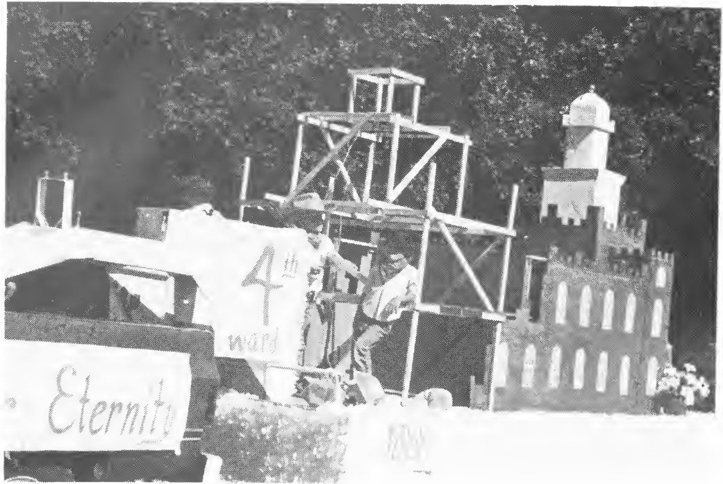
Replica of the construction of the Logan Temple--Fourth Ward
