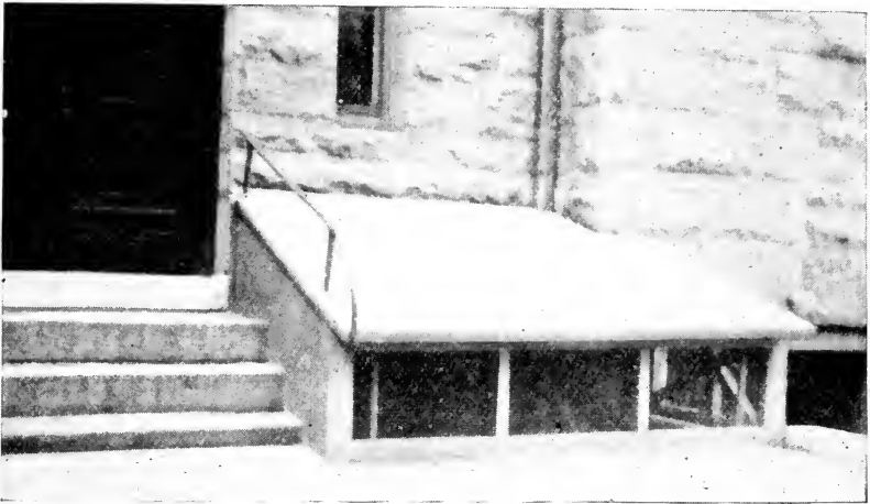
ILLUSTRATION 49. GROUND LEVEL AIR INTAKE OF THE FIRST BAPTIST CHURCH. IT SEEMS UNWISE TO TAKE AIR FROM DUST COVERED WALKS EVEN THOUGH IT IS WASHED BEFORE BEING SENT INTO THE ROOMS ABOVE
