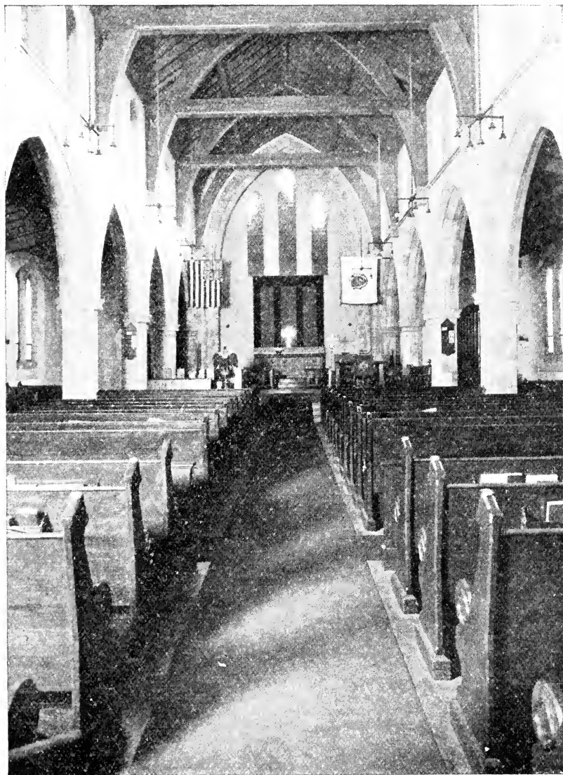
ILLUSTRATION 63. THE VERY ATTRACTIVE INTERIOR OF THE CHURCH AUDITORIUM OF THE ST. PAUL'S EPISCOPAL CHURCH
