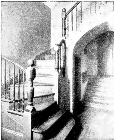
ILLUSTRATION 27. DANGEROUS WINDING STAIRS FOR PRIMARY CHILDREN. ST. PAUL'S EPISCOPAL CHURCH
