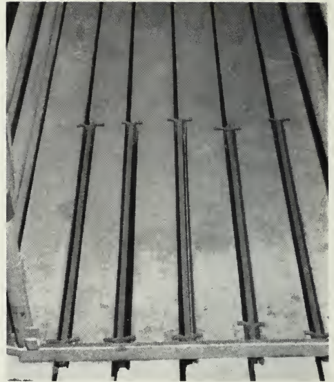
Figure 2. Totally slotted floors with steel slats (left) and concrete slats (right). The steel slats are 1 inch wide with \frac{1}{2} -inch spacings between slats; the concrete slats are 3 inches wide with \frac{1}{2} -inch spacings except at the rear of the pen, where spacings are wider (foreground). The iron rods are removed as soon as the pigs are old enough to cope with the wider openings.
