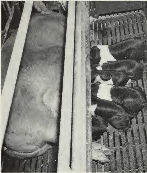
Figure 2. Totally slotted floors with steel slats (left) and concrete slats (right). The steel slats are 1 inch wide with \frac{1}{2} -inch spacings between slats; the concrete slats are 3 inches wide with \frac{1}{2} -inch spacings except at the rear of the pen, where spacings are wider (foreground). The iron rods are removed as soon as the pigs are old enough to cope with the wider openings.
