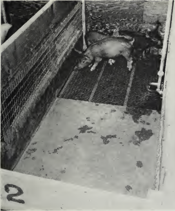
Figure 4. A nursery unit with a partially slotted floor. The concrete portion of the floor slopes toward the expanded metal-covered gutter. Electric heating units are in the floor near the feeder end of the pen. In a nursery unit with a totally slotted floor, environmental control is more critical.
