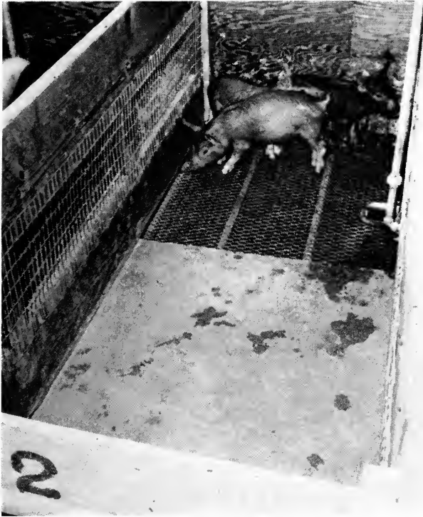
Figure 4. A nursery unit with a partially slotted floor. The concrete portion of the floor slopes toward the expanded metal-covered gutter. Electric heating units are in the floor near the feeder end of the pen. In a nursery unit with a totally slotted floor, environmental control is more critical.
