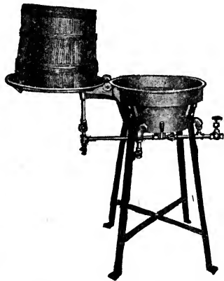
FIG. 33. — A butter tub paraffiner.
