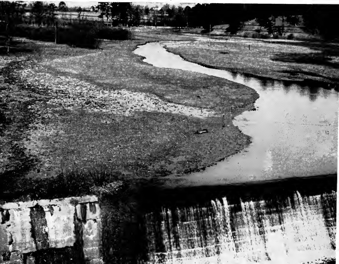
FIG. 51. In less than 20 years the Mayfair Mills power reservoir at Spartansburg, S. C., was filled with mud. This is not particularly hilly country, yet the farms in the watershed have contributed a lakeful of soil. The soil was lost; the investment in dam, reservoir, and powerhouse was lost; jobs were lost; recreational values were lost. What was gained? One mudhole.
