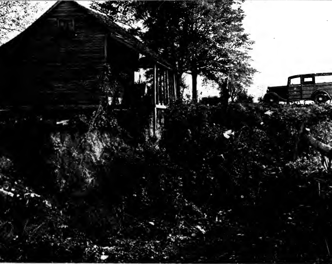
FIG. 44. This is the end result of breaking natural laws on the landscape. The gully will soon claim the house, then the road beyond. But, what good is a house or a road when the people have been exiled from the farm—sentenced by the court of natural justice. And, for how many generations will the children suffer for the incompetence of the father?
