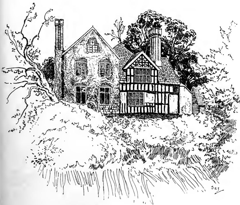
HARTON MANOR-HOUSE, SHROPSHIRE
