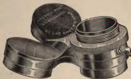
Fig. 11.—Triple Nosepiece.
