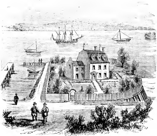
GOV. STUYVESANT'S HOUSE, ERECTED 1658, AFTERWARDS CALLED "THE WHITEHALL."
