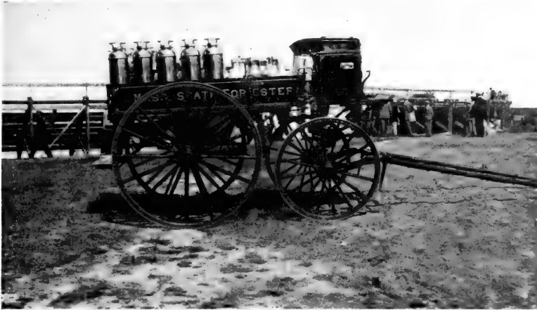
Fig. 58. — Special forest fire wagon; small size for one horse.
