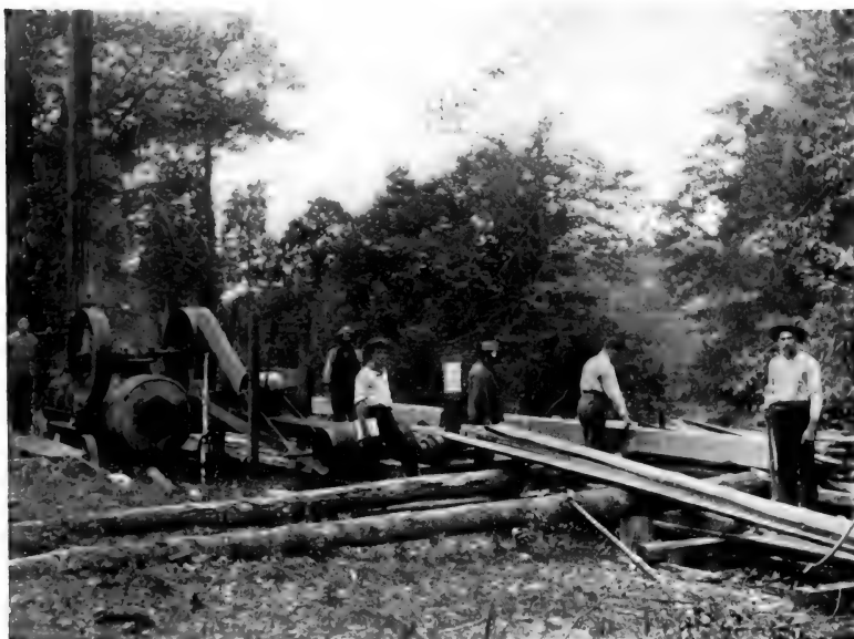
Fig. 60. — A portable sawmill of small capacity, such as is commonly used in southern New England.
