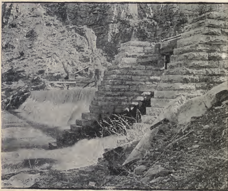
FIG. 32.—VIEW OF HIGHLINE CANAL WEIR.
