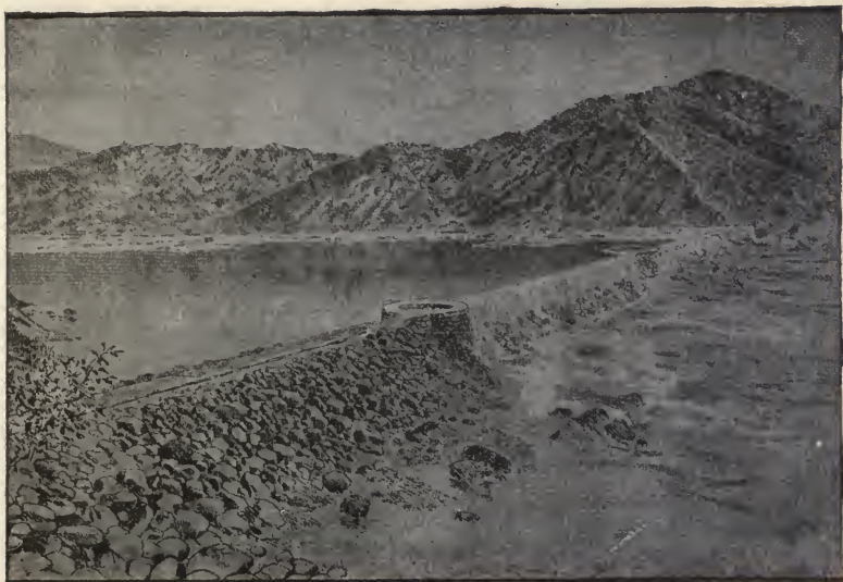
FIG. 76.—VIEW OF SAN FERNANDO SUBMERGED DAM.
