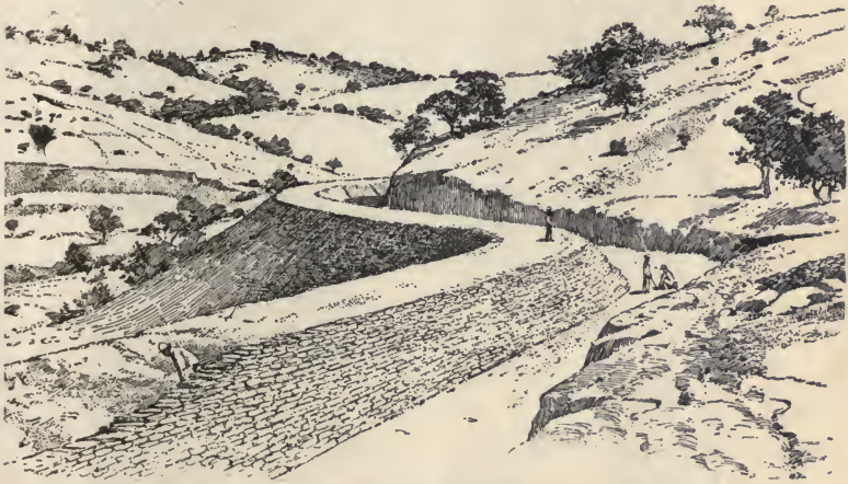
FIG. 10.—TURLOCK CANAL. VIEW OF SIDEHILL WORK.
