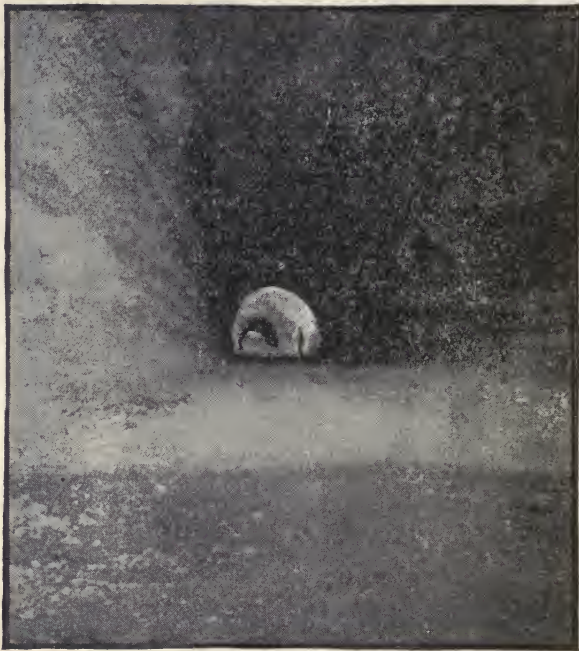
FIG. II.—TURLOCK CANAL. VIEW IN TUNNEL.
