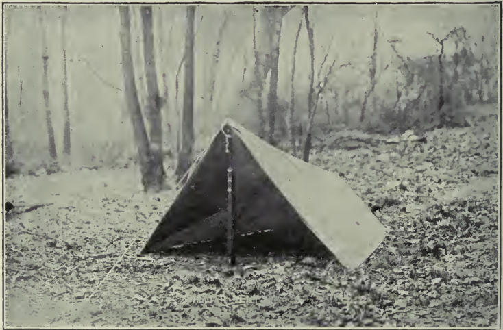
FIG. 186.—Shelter tent, pitched on rifle and bayonet.
