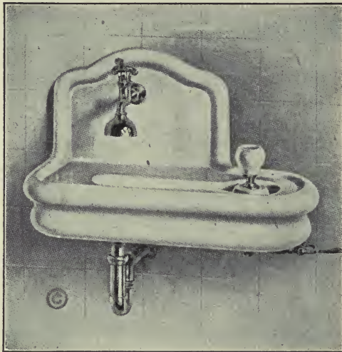
FIG. 38.—Wash-hand basin, with sanitary bubbling cup at the right, which flows when the lever below is pressed down. (American Medical Association Building.)
