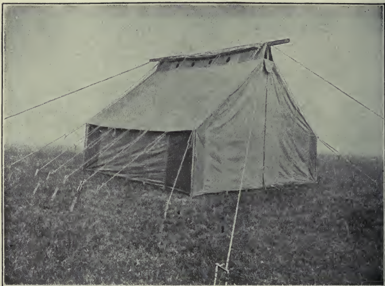
FIG. 194.—Hospital tent, tropical, showing ventilation of attic.
