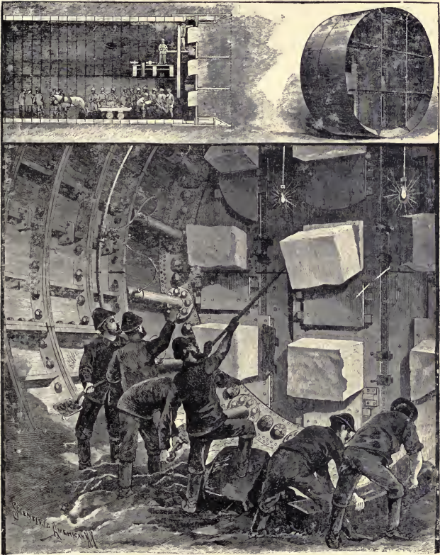
FIG. 273.—The Hydraulic Shield.
