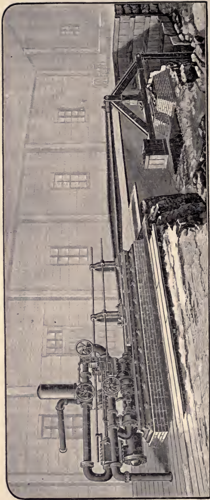
FIG. 148.—Hydraulic Pumping-engine.
