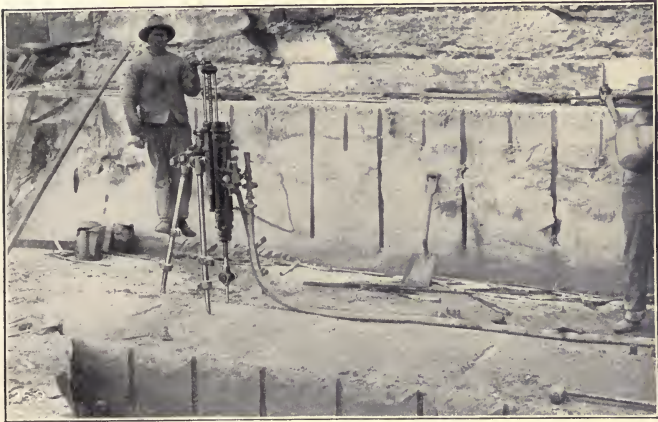
FIG. 306.—Blocking out Dimension Stone.
