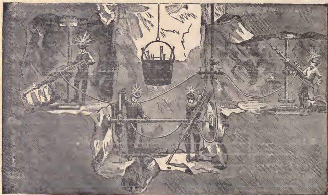
FIG. 305.—The Column Support for Drills.
