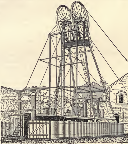
FIG. 81.—A Steel Head-frame at a Bituminous Colliery.
