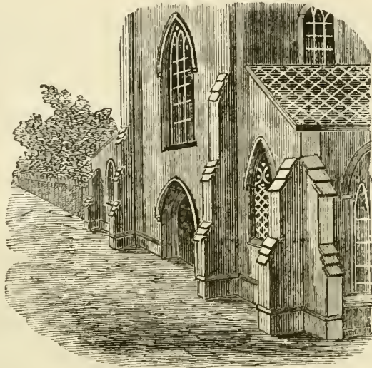
WEST FRONT OF ST. MARK'S CHURCH, Philadelphia.—Exaggerated perspective of short focus lens.
