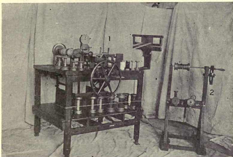
FIG. 14.—1. Edge-warping machine and anchor bobbins. 2. Hand-drive edge take-off machine.
