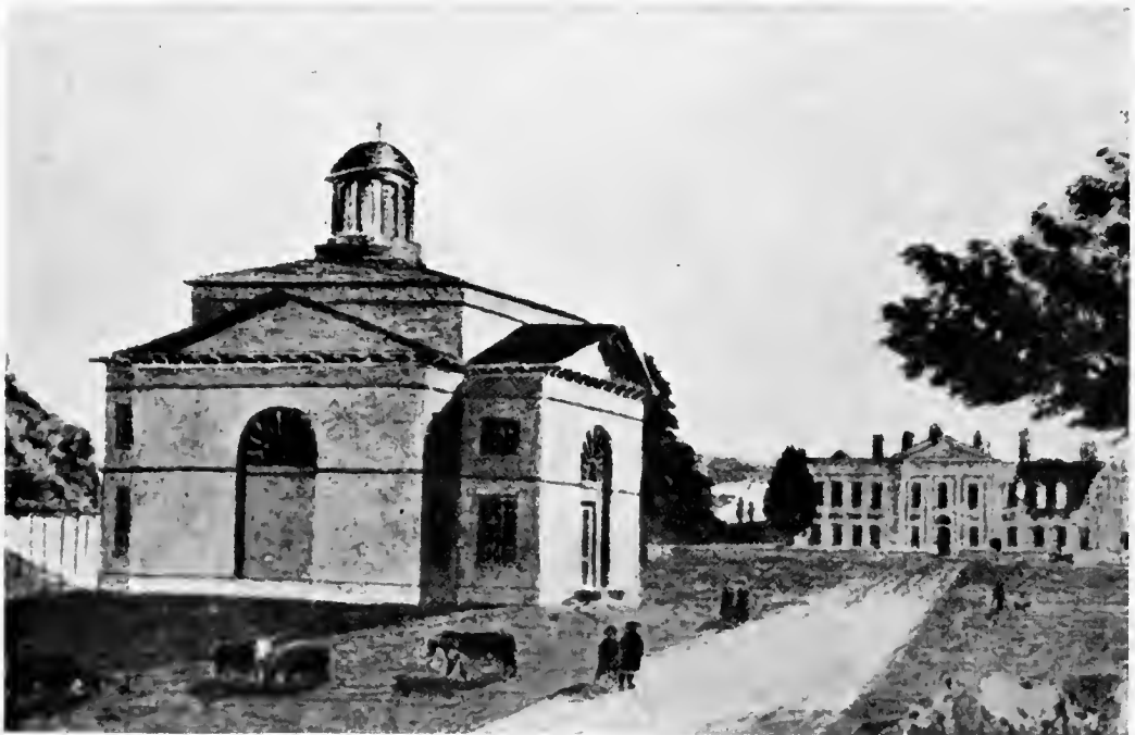
EARLY VIEW OF ST. JOHN'S CHURCH
