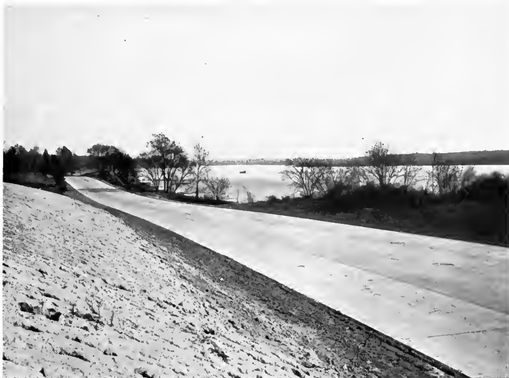
MOUNT VERNON MEMORIAL HIGHWAY, NORTH OF LITTLE HUNTING CREEK
