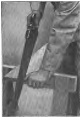
Fig. 6—Starting the Rip Saw
