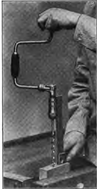
Fig. 71a—Squaring Auger Bit with Try Square
