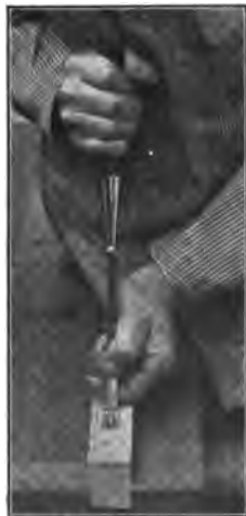
Fig. 70j—Bevelling to End Lines of Mortise
