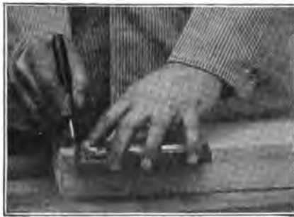
Fig. 39g—Knife and Square in Position for Drawing Line
