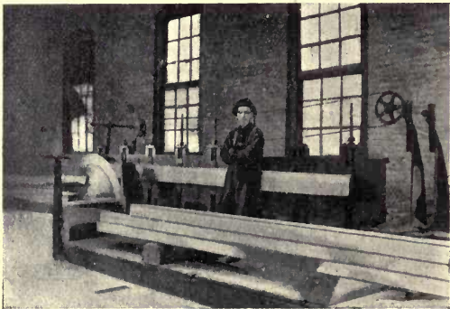
FIG. 7.—VENEER SAW AND FLITCHES.
