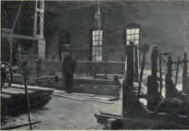
FIG. 4.—BAND SAW CARRIAGE.
