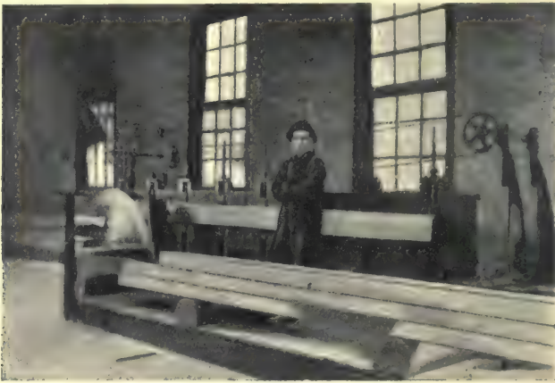
FIG. 7.—VENEER SAW AND FLITCHES.
