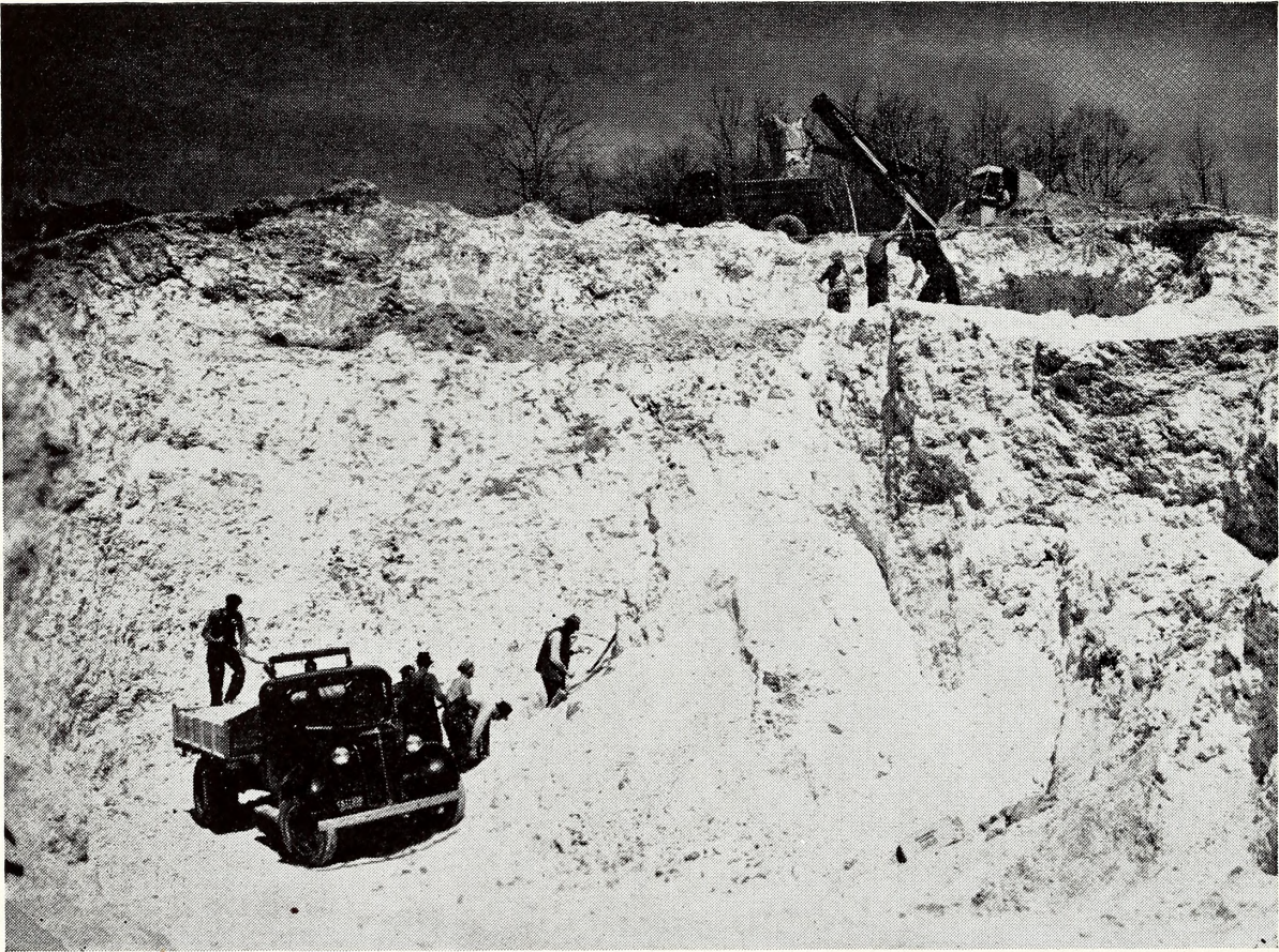
Figure 5. A Mine of Harris Clay Co., near Spruce Pine, N. C.
