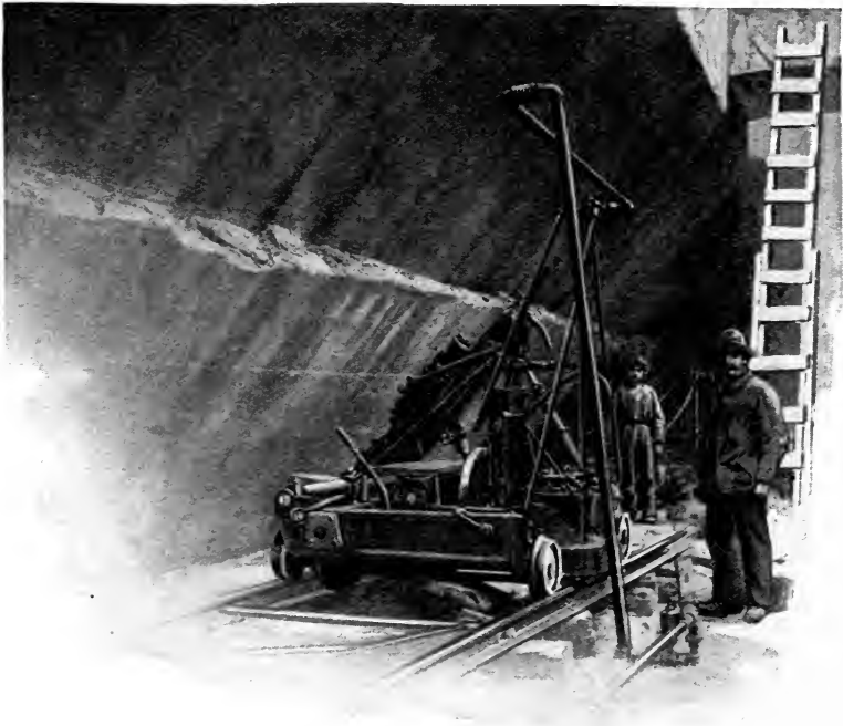
UNDERCUTTING WITH THE SULLIVAN CHANNELLER.
