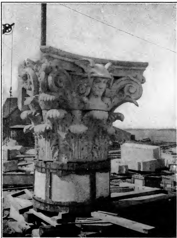
ARCHITECTURAL CARVING EXECUTED WITH INGERSOLL PNEUMATIC APPLIANCES, NEW YORK, U.S.A.
