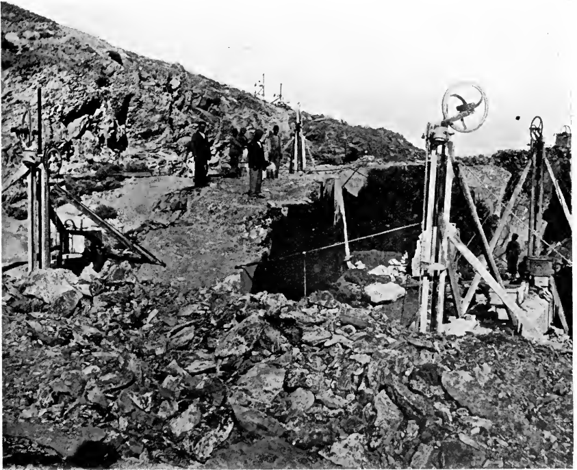
THE WIRE SAW IN OPERATION AT TINOS, GREECE.
