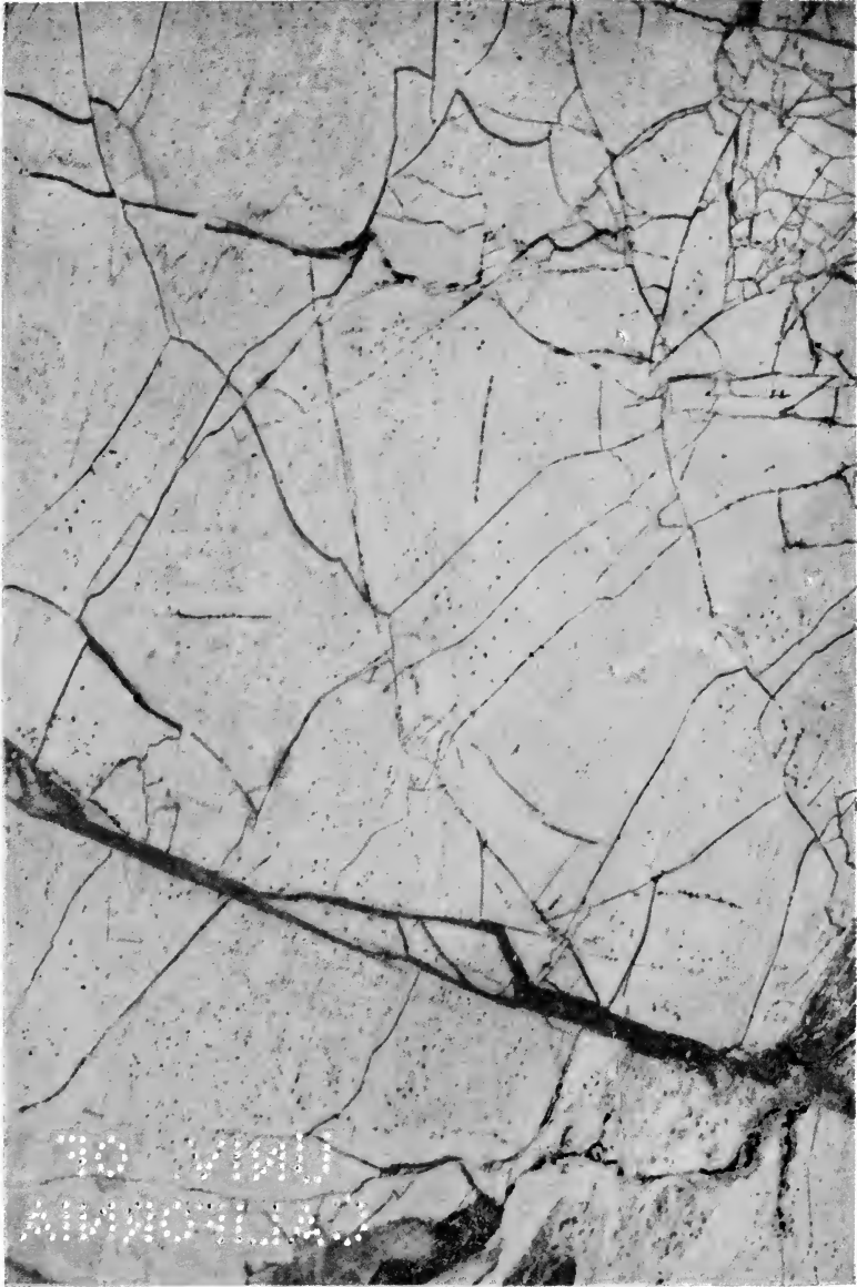
Fig. 1. Cracks in the rock surface. [The face p. 199.]
