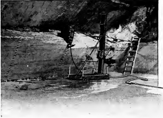
THE GADDER AT WORK ON UNDERCUT SLOPE.
