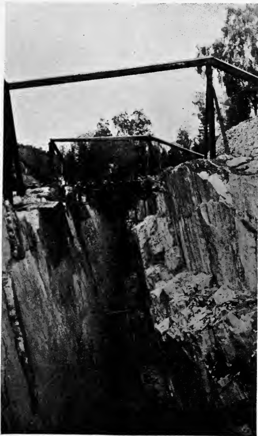
A SWEDISH MARBLE QUARRY, MARMORBRUKET, NEAR NORRKÖPING.
