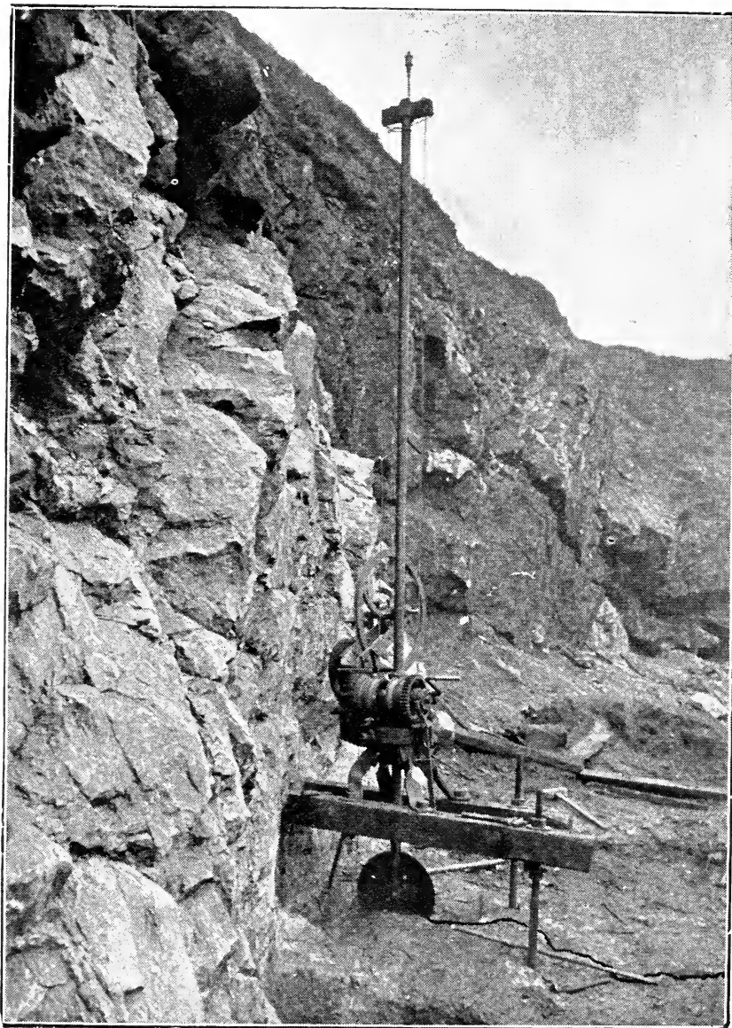
THE PENETRATING PULLEY OPERATING AT BERGNIORNY, BELGIUM.
