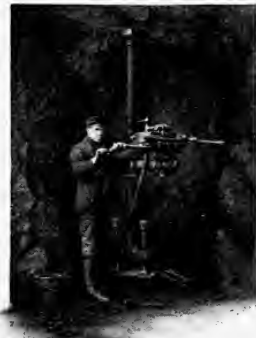
INGERSOLL DRILL MOUNTED ON COLUMN.
