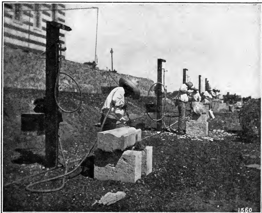
MASONS WORKING WITH PNEUMATIC TOOLS, HUEYAPAM, MEXICO.
