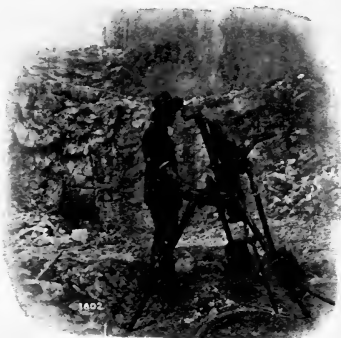
INGERSOLL DRILL MOUNTED ON TRIPOD.
