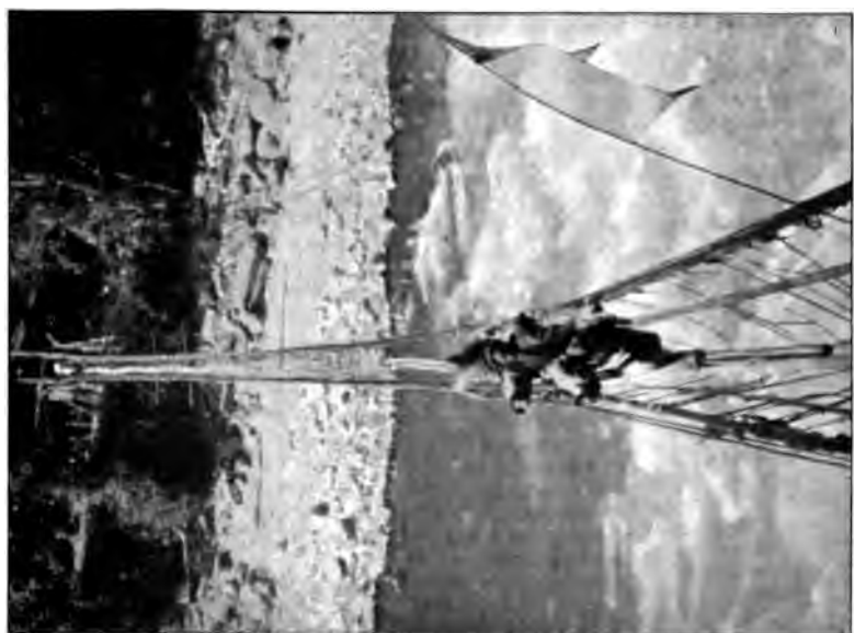
Showing construction of Cane Bridge—the bamboos forming the footway lie loose within loops made of strands of bark.
