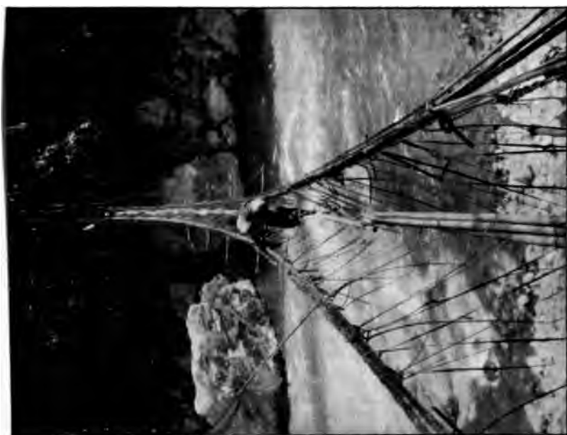
Showing construction of Cane Bridge—the bamboos forming the footway lie loose within loops made of strands of bark.
