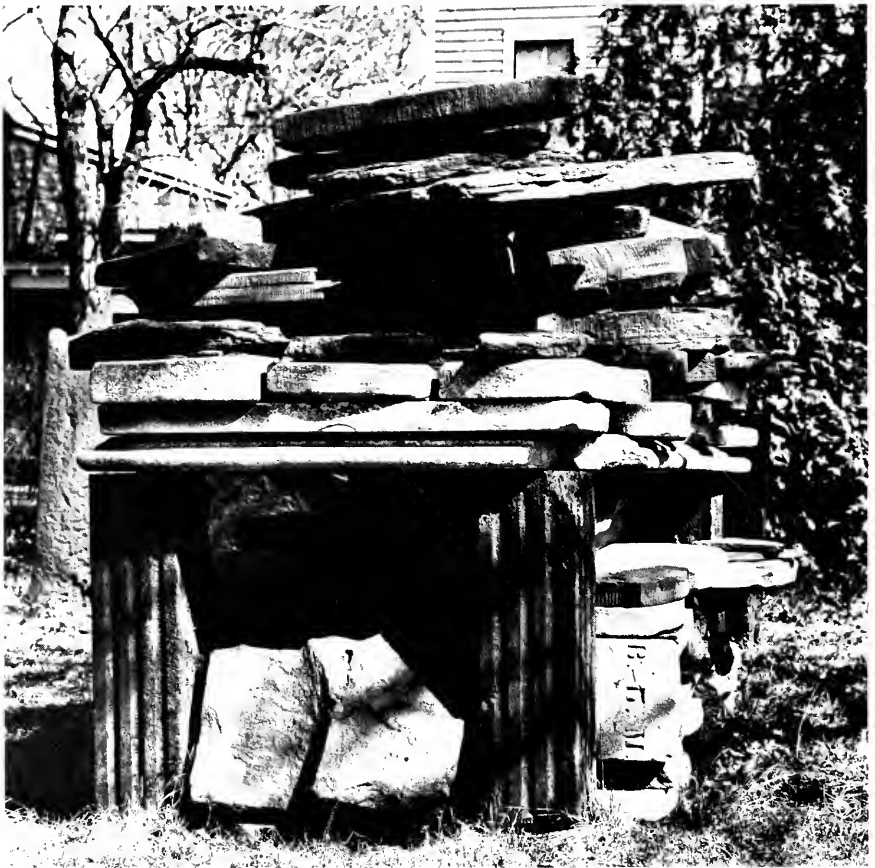
Springfield, N.J. In a neglected yard for Revolutionary War dead, broken gravestones are piled randomly on top of and under a table stone. While this practice avoids stone loss, it is contrary to sound gravestone conservation.
