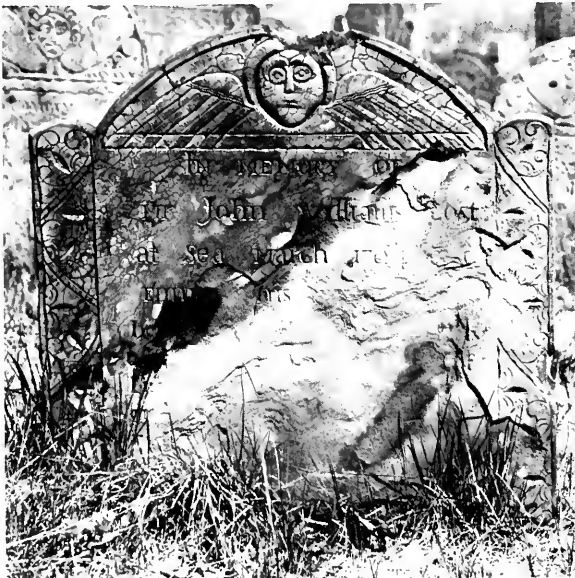
Norwichtown, Conn. Overall fissures in stone fronts bring about crumbling and erosion during the terminal phase of eradication caused by the freeze/thaw cycle.
