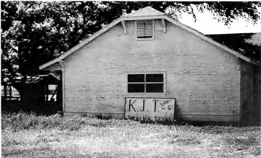
Fig. 13. Abandoned Czech Catholic Union building, Dubina, Texas.
