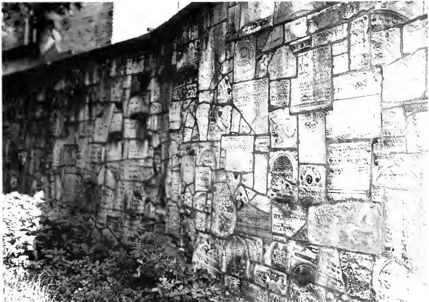
Fig. 3. Wall of Remu Cemetery, Cracow, Poland. The wall was constructed with headstones the Nazis removed from the cemetery or damaged.
