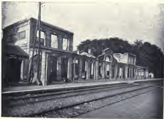
INTERIOR OF THE BURNT STATION (Sept. 1914)
