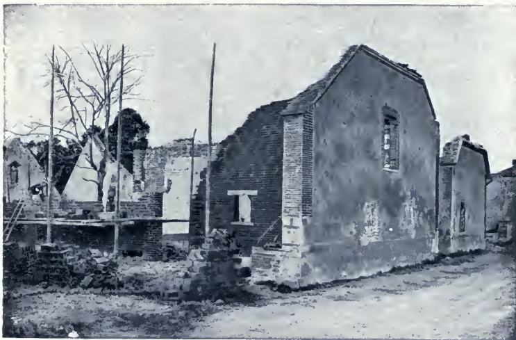
HOUSES BEING REBUILT AT MORAINS
