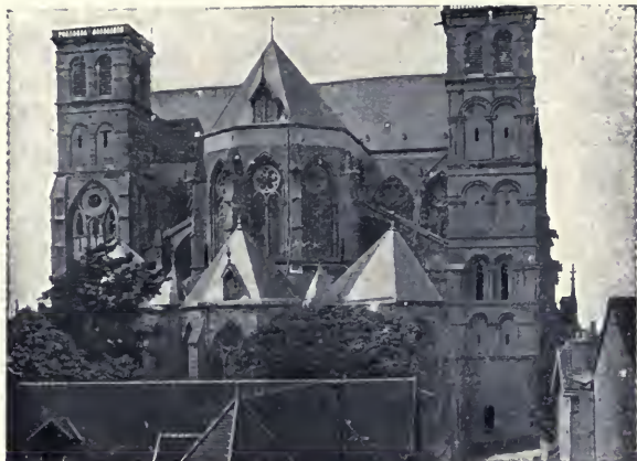
APSE AND TRANSEPT OF THE CATHEDRAL
