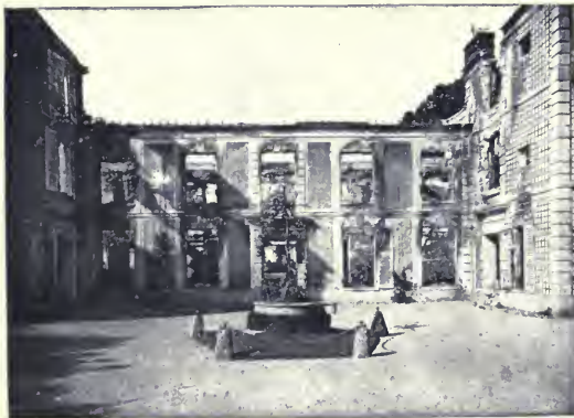
BURNT BUILDING 17, FAUBOURG ST. MARTIN
