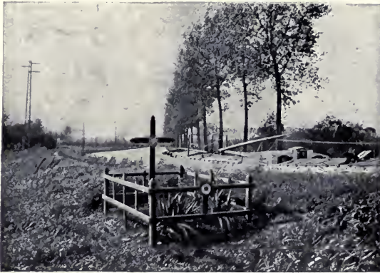
THE CANAL AT PARGNY (looking westwards)
