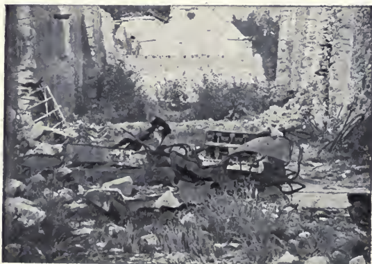
DEBRIS OF THE CASTLE MOTOR-CAR
