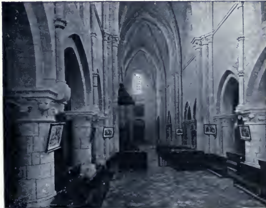
NAVE OF VOULTON CHURCH
