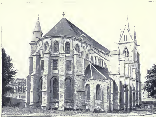
THE CHURCH SEEN FROM THE ROAD
