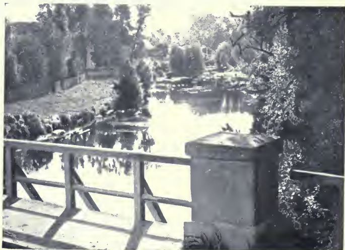
BRIDGE OVER THE MORIN
