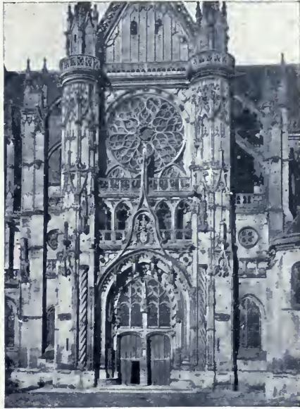
THE CATHEDRAL SOUTH FAÇADE OF TRANSEPT
