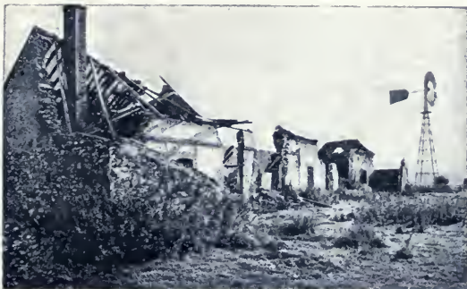
WINDMILL WATER PUMP AT LA VILLENEUVE
