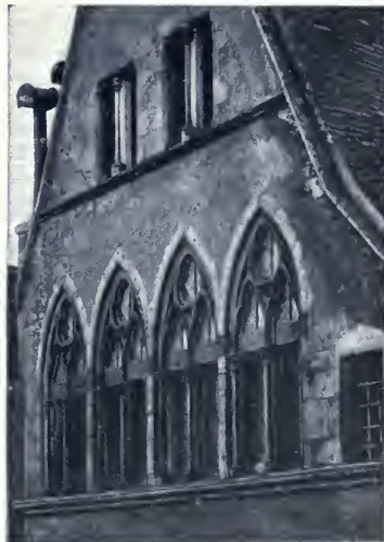
WINDOWS OF THE HOTEL VAULTUISANT
