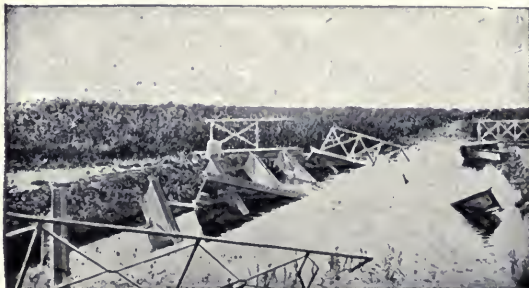
DESTROYED BRIDGE OVER THE MORIN
