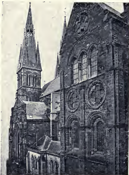
PORCH AND SOUTH TRANSEPT OF NOTRE-DAME
