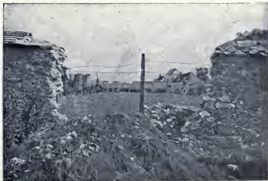
BREACH IN THE SOUTHERN WALL OF THE CASTLE
