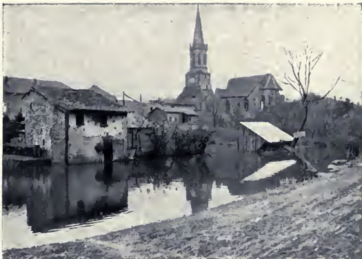
VIEW OF BAUZÉE
