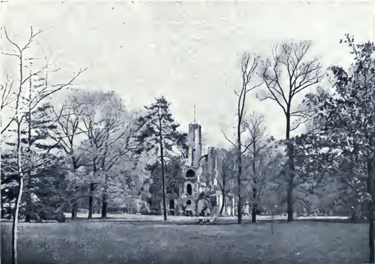
RUINS OF THE CHURCH SEEN FROM THE ROUTE DES ÉTANGS
