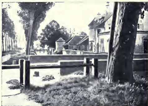
BRIDGE OVER AN ARM OF THE MORIN
