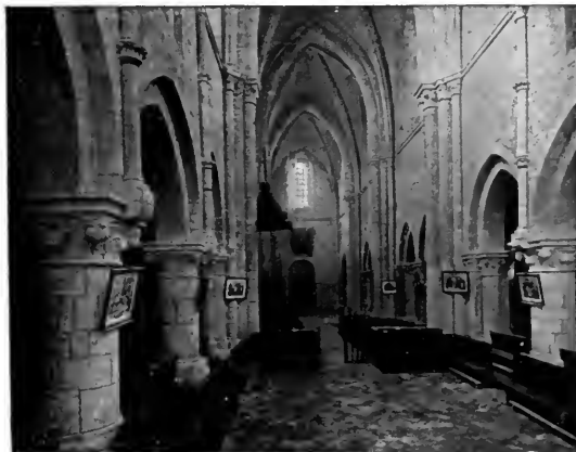
NAVE OF VOULTON CHURCH
