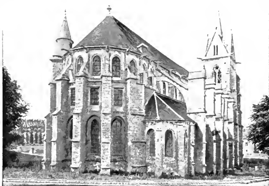
THE CHURCH SEEN FROM THE ROAD
