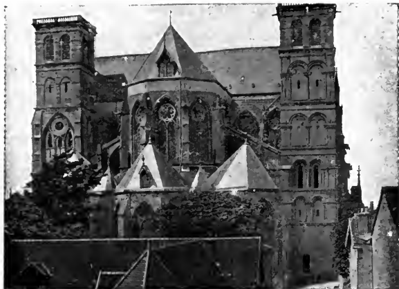
APSE AND TRANSEPT OF THE CATHEDRAL
