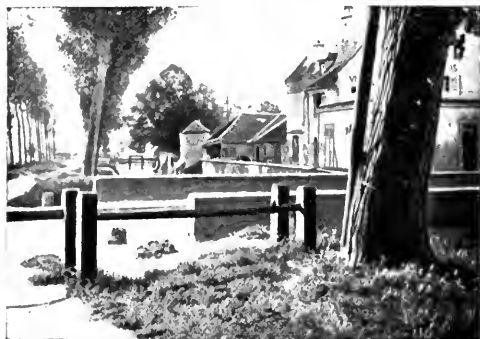
BRIDGE OVER AN ARM OF THE MORIN
