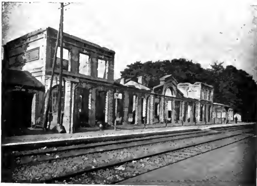
INTERIOR OF THE BURNT STATION (Sept. 1914)
