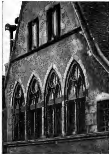
WINDOWS OF THE HOTEL VULUISANT
