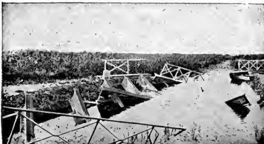
DESTROYED BRIDGE OVER THE MORIN
