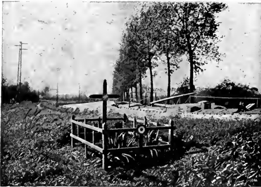
THE CANAL AT PARGNY (looking westwards)
