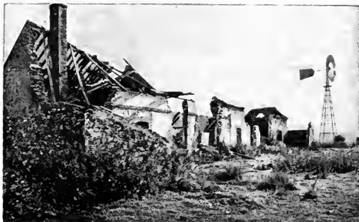
WINDMILL WATER PUMP AT LA VILLENEUVE
