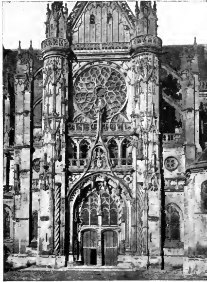
THE CATHEDRAL SOUTH FAÇADE OF TRANSEPT
