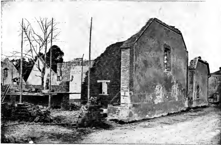
HOUSES BEING REBUILT AT MORAINS
