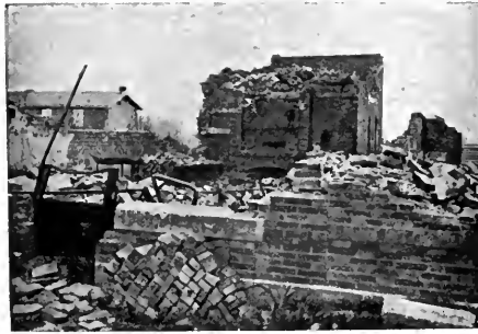
HOUSES DESTROYED IN HUIRON
