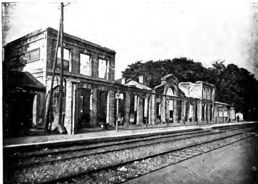
INTERIOR OF THE BURNT STATION (Sept. 1914)
