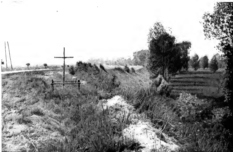
TRENCH NEAR THE SOMME
