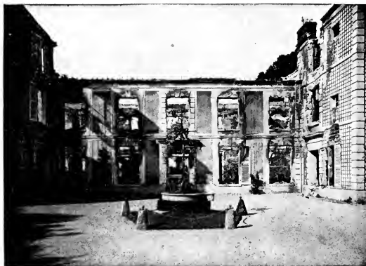
BURNT BUILDING 17, FAUBOURG ST. MARTIN
