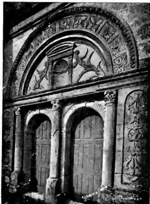
DOORWAY OF DAMMARTIN CHURCH
