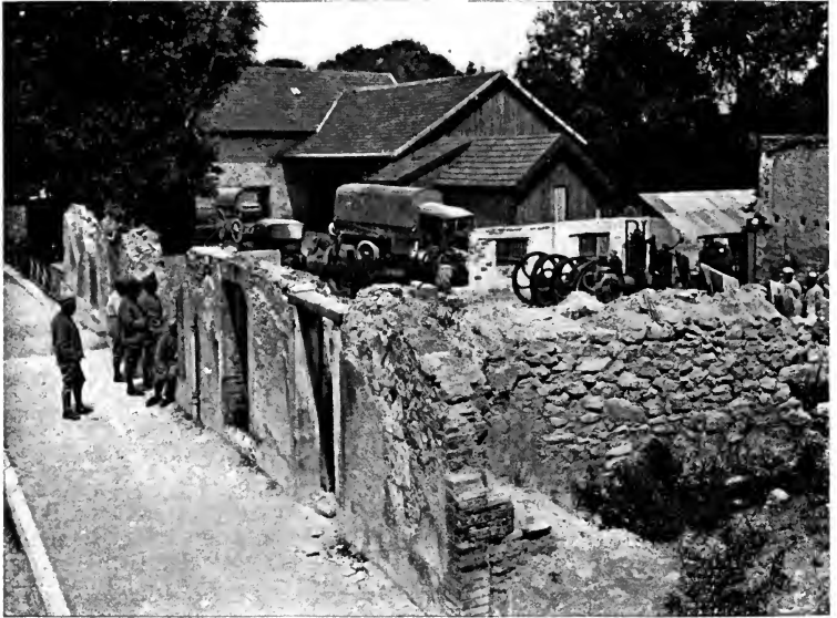
RUINS OF THE ELECTRIC POWER STATION
