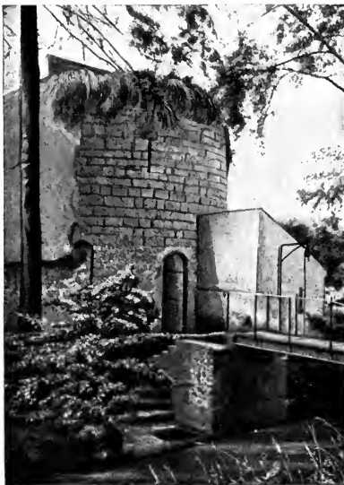
TOWER BELONGING TO THE OLD WALL
