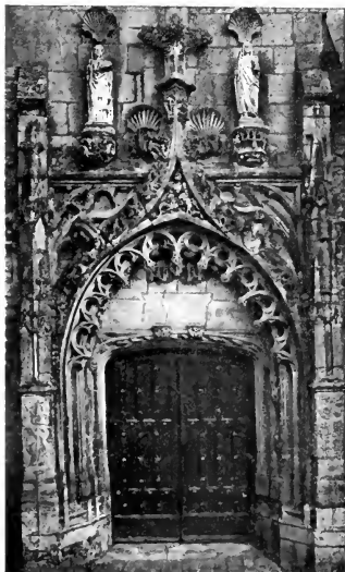
DOORWAY AT SAINTE-CROIX
