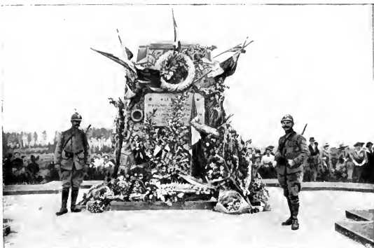
MONUMENT OF THE FOUR ROADS
