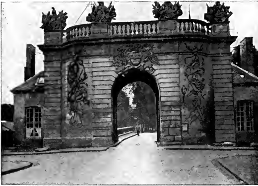
GATEWAY OF BRIDGE
