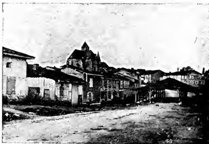
VIEW OF CHEMINON (looking west)
