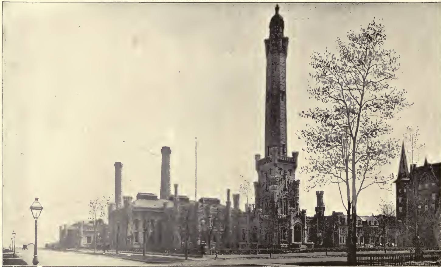
NORTH SIDE PUMPING STATION.
