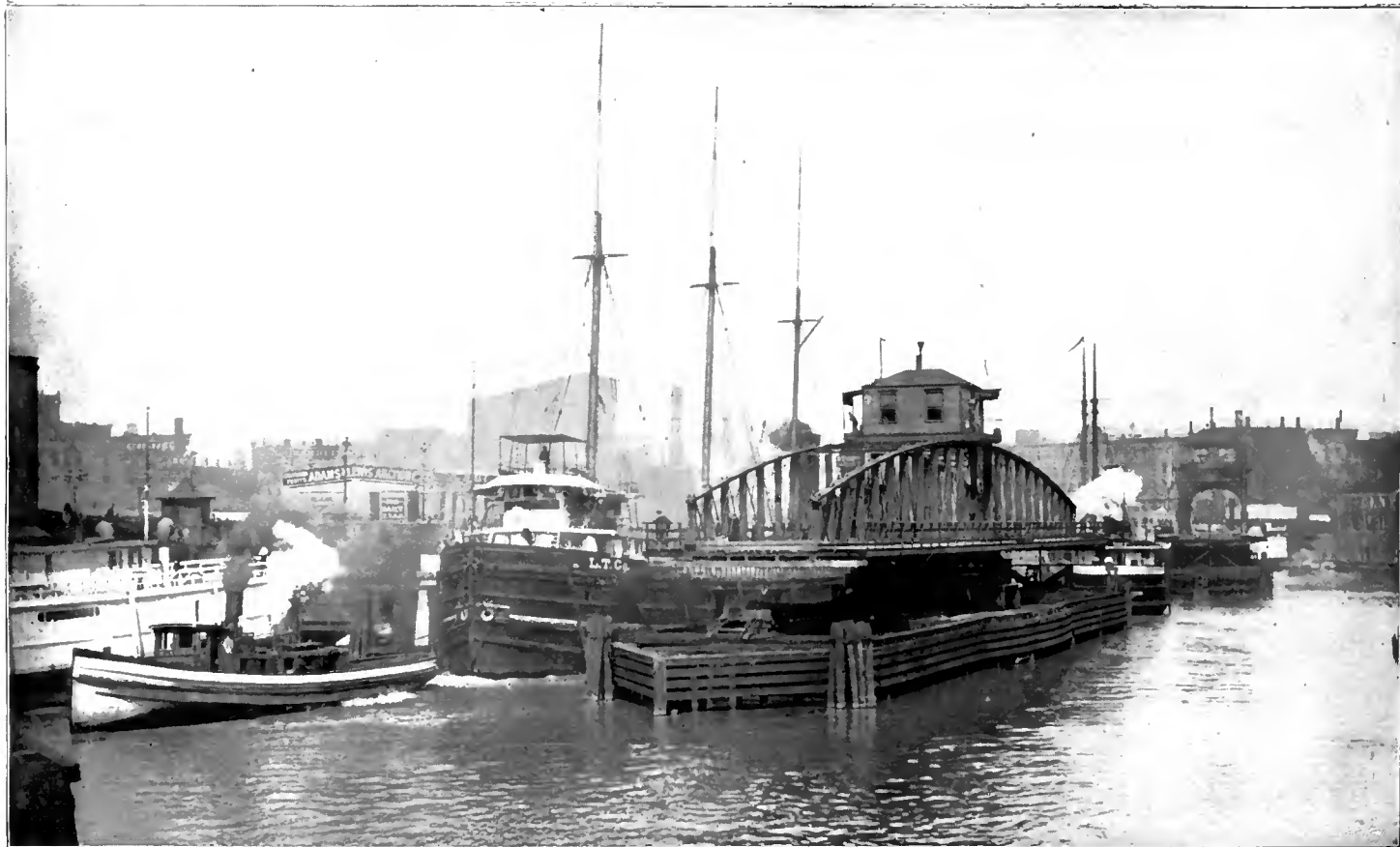
CHICAGO RIVER, CLARK STREET BRIDGE LOOKING WEST.
