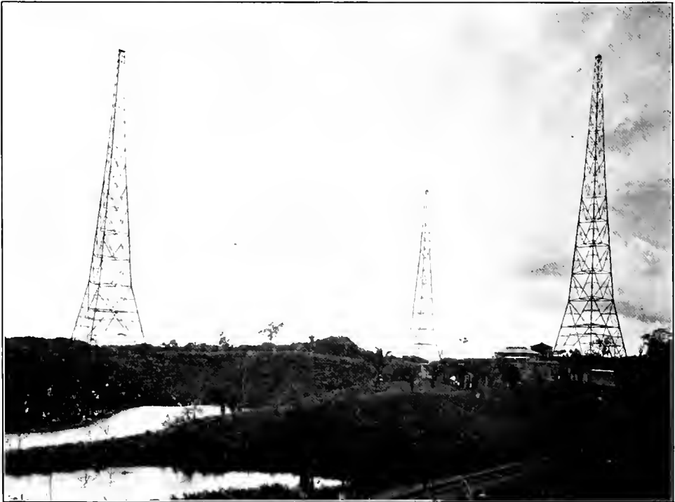
THE DARIEN RADIO TOWERS AT PANAMA
