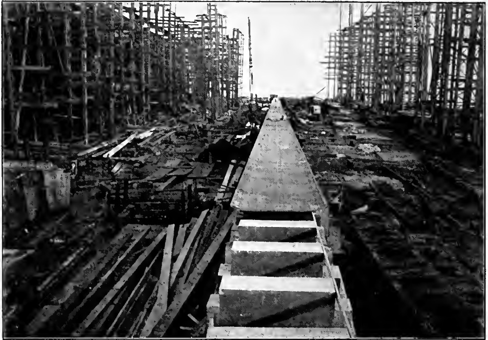
LAYING A BATTLESHIP'S KEEL AT THE FORE RIVER SHIPYARDS
