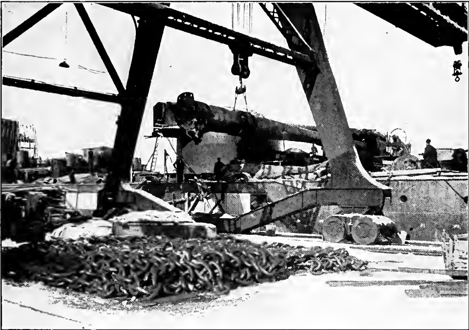
INSTALLING HER 14-INCH GUNS
