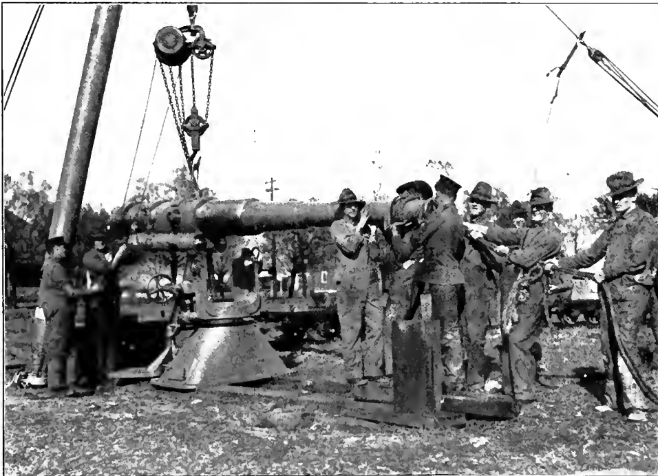
ADVANCE BASE PRACTICE IN MOUNTING 6-INCH GUN
