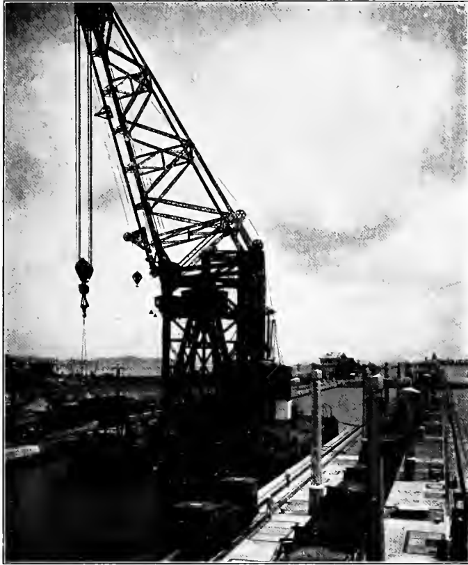
THE FLOATING CRANE "HERCULES" IN GATUN LOCKS
