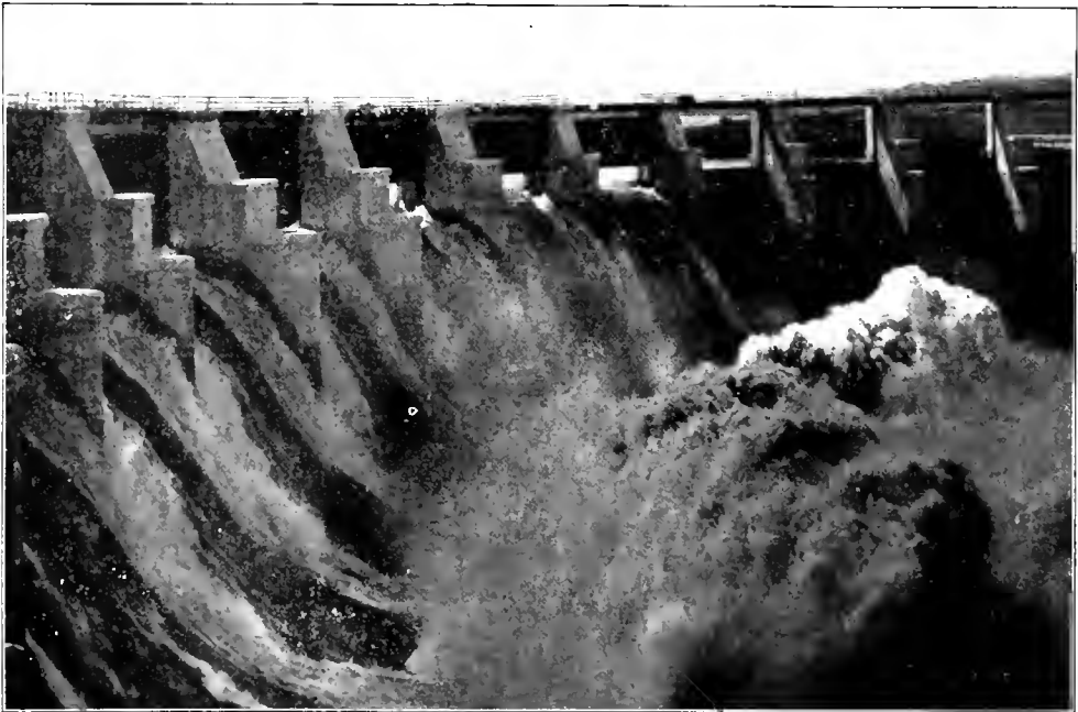
THE GATUN SPILLWAY WITH SEVEN GATES OPEN
