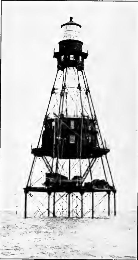
THE SCREW PILE STATION IN FLORIDA WATERS
