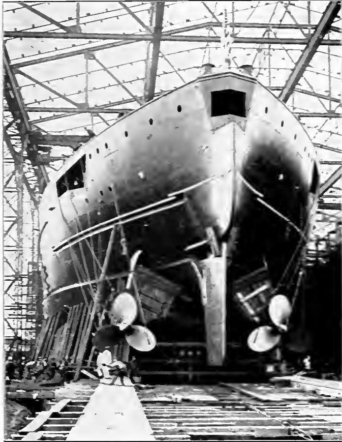
THE STERN VIEW WHEN READY FOR LAUNCHING
