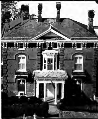
Is it just us, or does everyone have a soft spot for the charming grace of Rose Terrace — now in great need of renovation?
