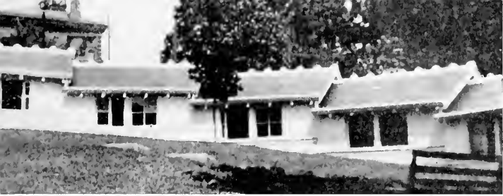
A section of the covered way (Rose Terrace just visible behind it) — going up hill and down!
