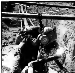
7/7/06 – A welder works in the front campus trench
