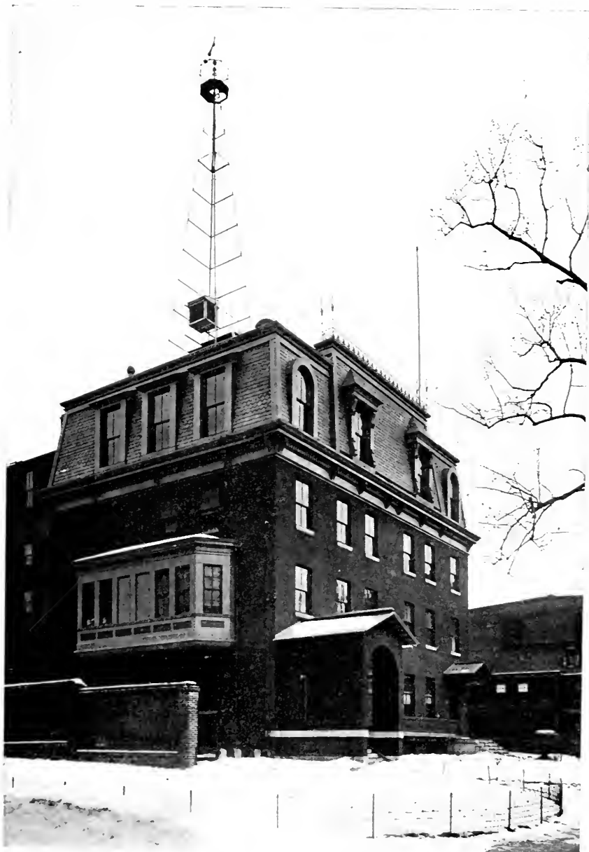
OFFICE OF THE U. S. WEATHER BUREAU, JOHNS HOPKINS UNIVERSITY, No. 532 NORTH HOWARD STREET. MARYLAND STATE WEATHER SERVICE.
