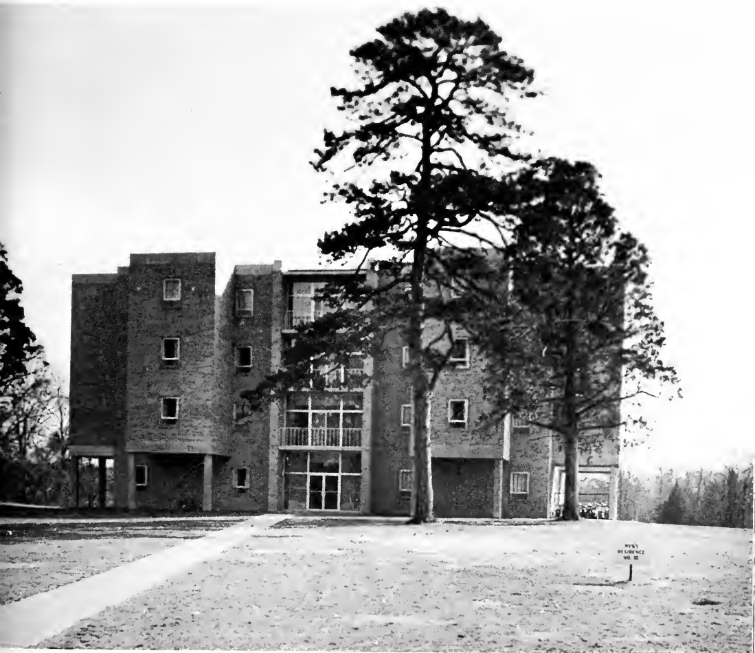
MEN'S RESIDENCE Erected 1966
