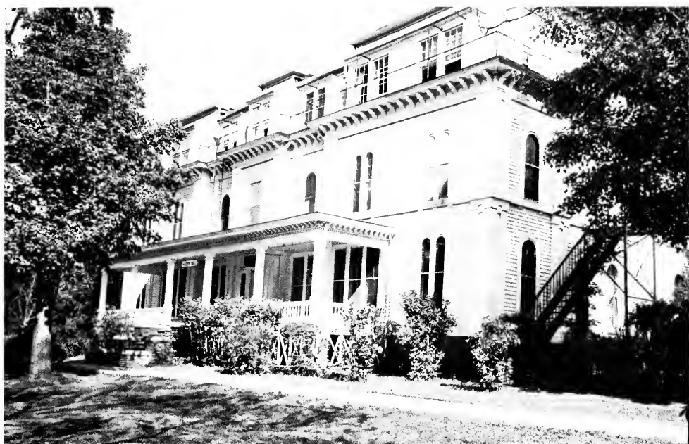
BALDWIN HALL Erected 1871; removed 1968
