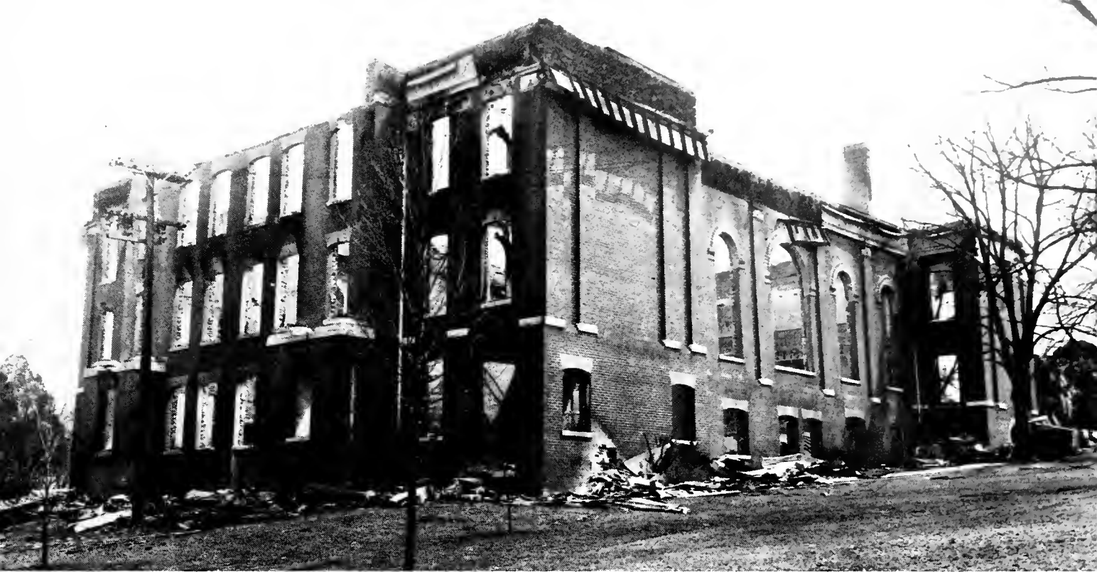
After the Chapel burned and before the walls fell.
