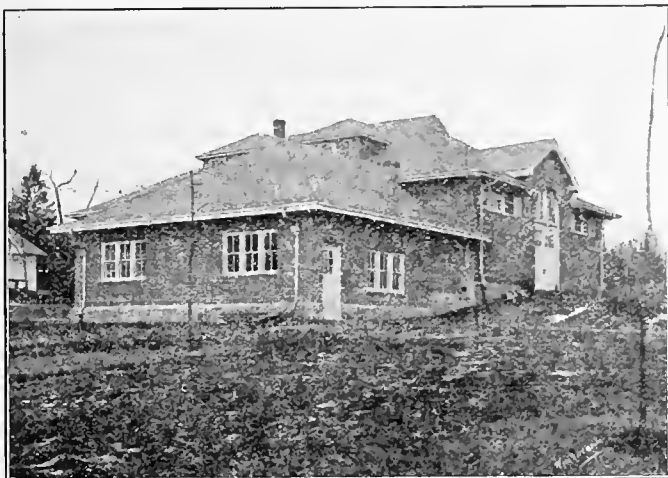
New Abattoir Addition to Grinnell Arena which was recently completed
