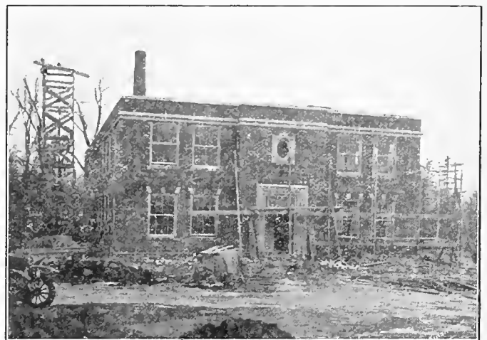
New Horticultural Manufactures Building located west of Flint Laboratory
